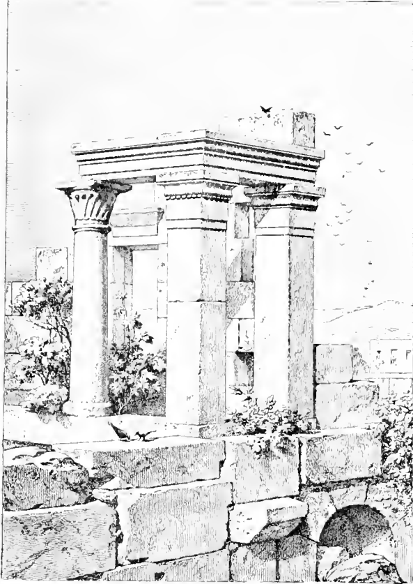
PILLAR: SQUARE AND ROUND ONES (COMMONLY CALLED PIERS AND COLUMNS), KOKANAYA, SYRIA; 5TH CENTURY A.D.
